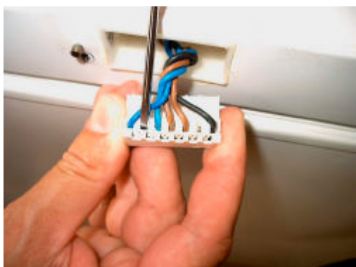
4. Open the clips of the fixing cover of the connector
